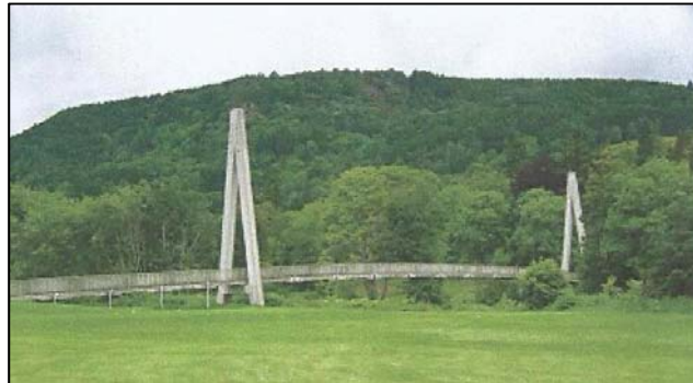
Figure 2. Aberfeldy Golf Course suspended footbridge.
