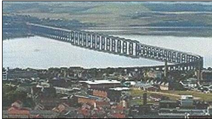
Figure 4. Tay rail bridge today.
