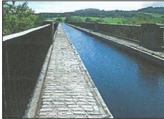
Figure 13. Avon Aqueduct from above.
