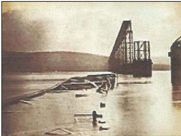
Figure 5. Picture of the Tay rail bridge the day after its failure.
